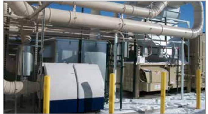
The MultiAir® blowers are weatherproof and have low noise level
